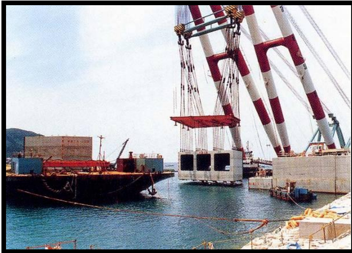
Installation of Outlet of Seawater (May 1985) (19m width, 18m 3 /sec)
