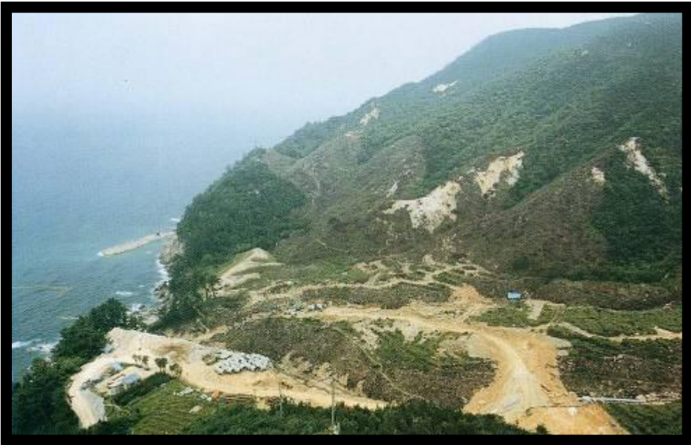
Initial Access Road
